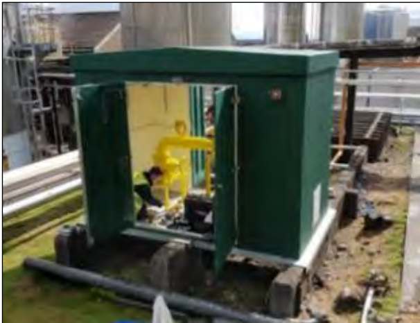
Final 2 bar to 200 mbar Regulator
