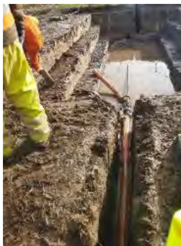
HDD of Soluforce Pipeline
