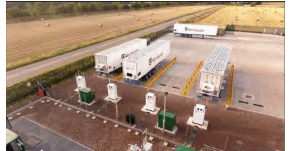
Bio-CNG trailers being Filled
