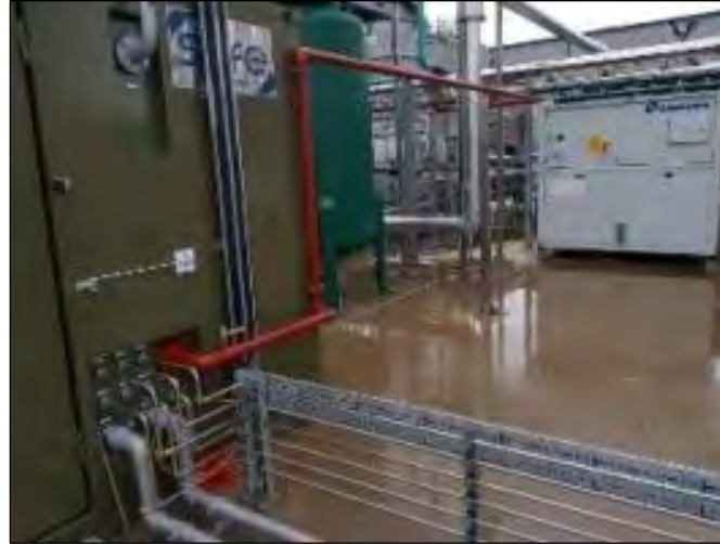
Inlet to Compressor
