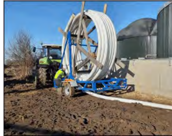
75 bar Soluforce Pipeline
