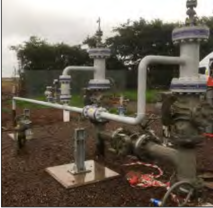
Connection at 85 Bar Block Valve
