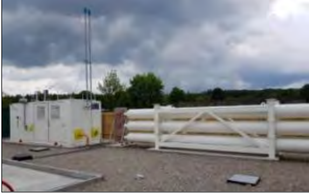
PRMS (250 – 2barg) and Bio-CNG Storage
