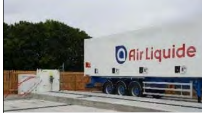
Offloading Cabinet and Bio-CNG Trailer
