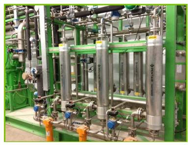
Membranes used to separate the CO2 from the CH4
