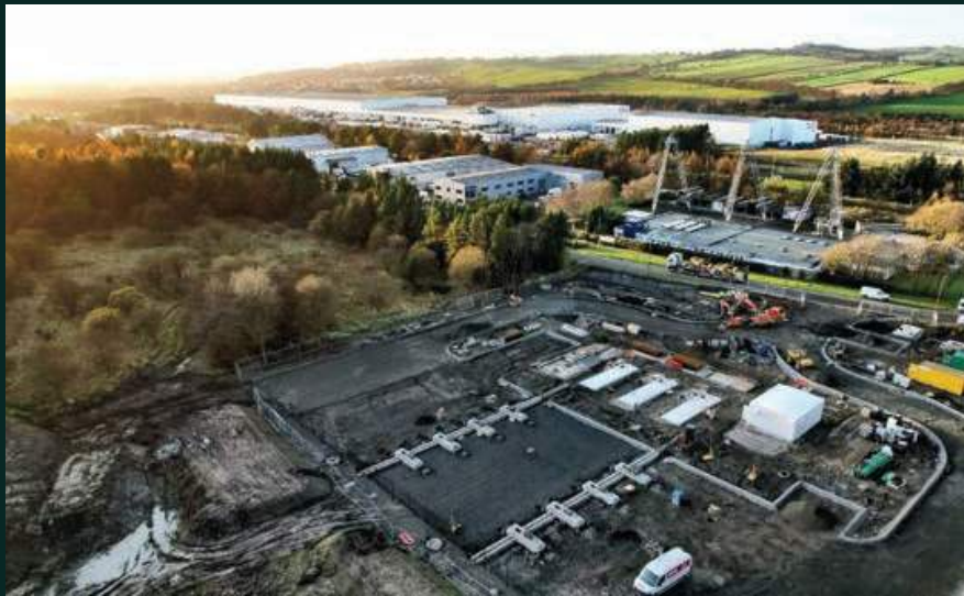
Well underway with concrete being poured
