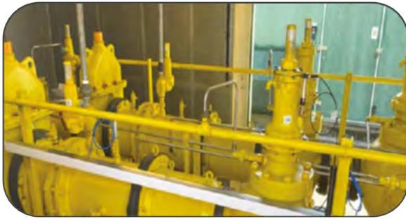
Installation of flow metering across our network
