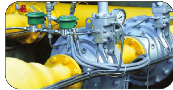
Installation of smart pressure control equipment
