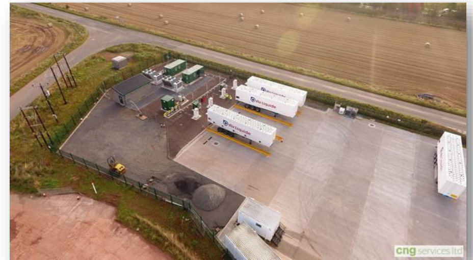
Air Liquide Fordoun Mother Station – shows trailer filling bay
