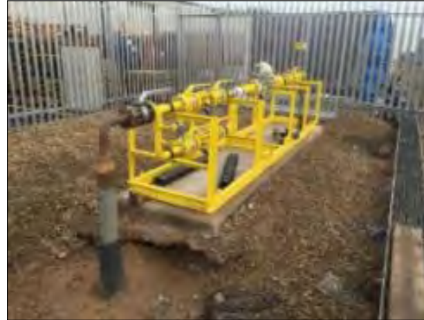
First Unregulated Gas Meter for Bio-CNG
